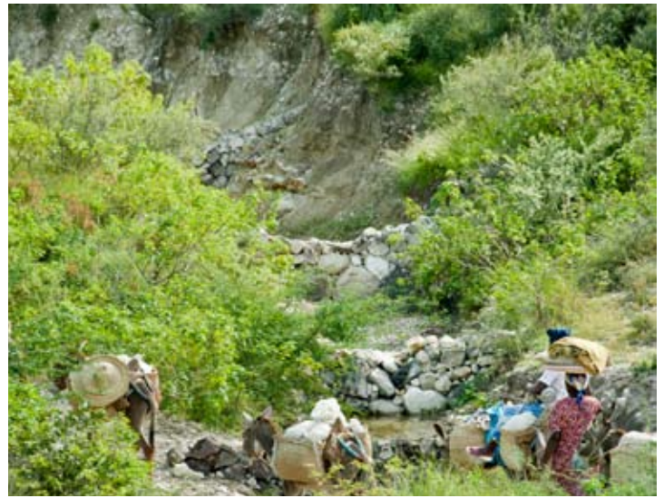
Ravine barrages prevent floods from swamping the village below. Topsoil and water are retained.
