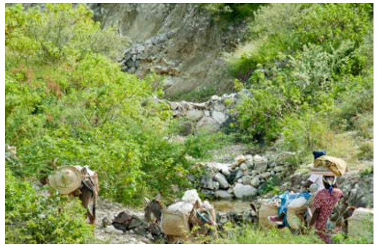
Ravine barrages prevent floods from swamping the village below. Topsoil and water are retained.
